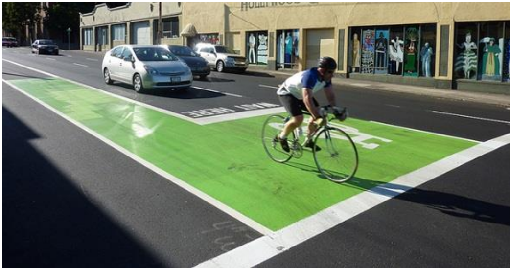
An intersection in Portland, OR utilizing a bike box at the head of a traffic lane. Source: Otrec
