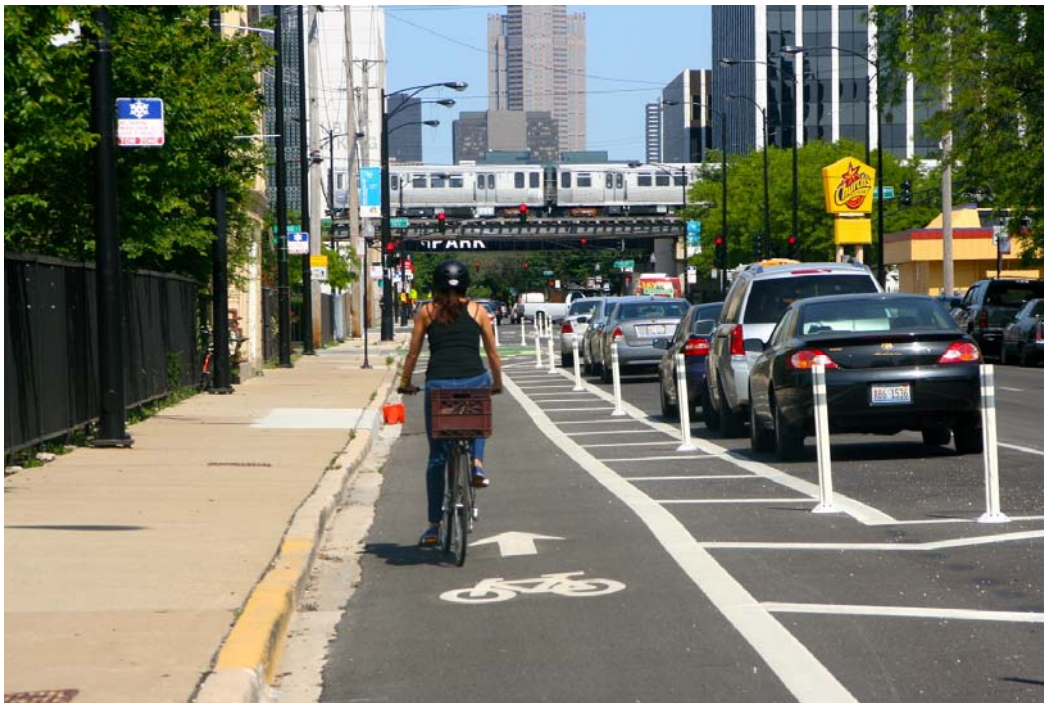
A one-way protected lane utilizing bollards to create separation for bicyclists on Kinzie St. in Chicago, IL. Source: People for Bikes
