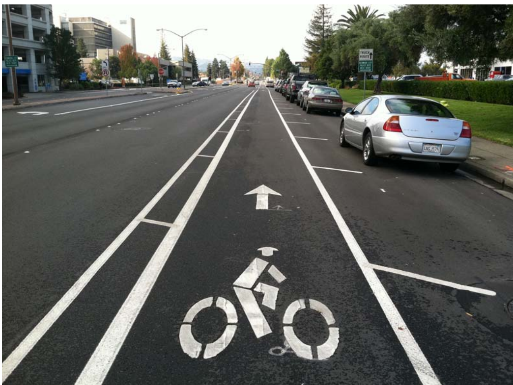
A buffered bike lane that utilizes a buffer zone on both the travel lane and parking lane sides in Kansas City, KS. Source: Bike Walk KC
