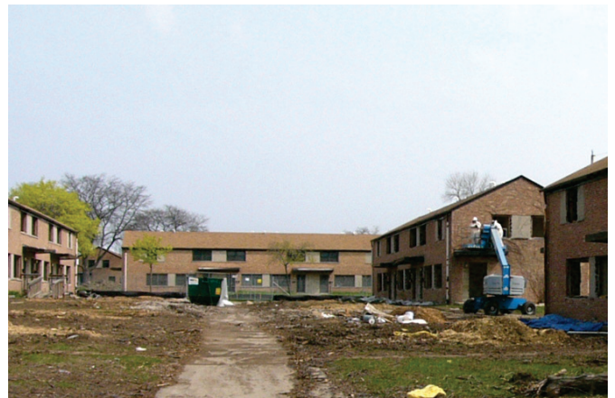
Westlawn Demolition and Renovations Underway
