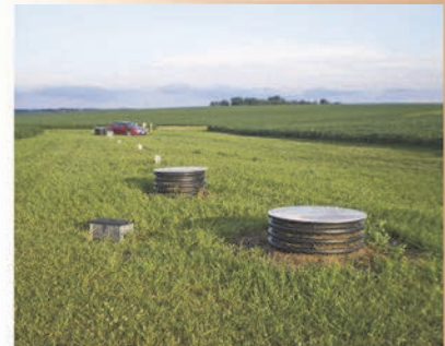
Figure 7. Woodchip bioreactor after installation; circular sumps and PVC wells used for research monitoring (Northeast Iowa Research and Demonstration Farm)
