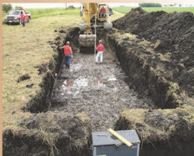
Figure 4. Excavation for a bioreactor installation (courtesy of the Iowa Soybean Association Environmental Programs and Services)
