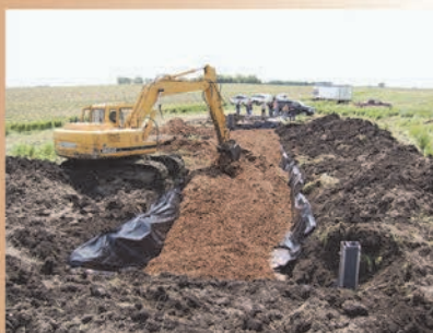
Figure 5. Filling an excavation with woodchips for a bioreactor installation (courtesy of the Iowa Soybean Association Environmental Programs and Services)
