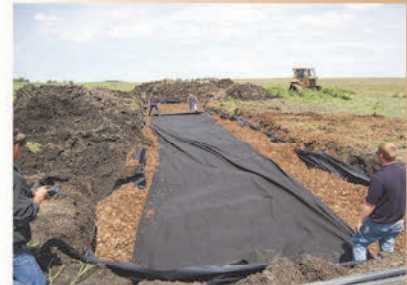
Figure 6. Covering the woodchips with a geo-textile fabric before laying the soil cover at a bioreactor installation (courtesy of the Iowa Soybean Association Environmental Programs and Services)
