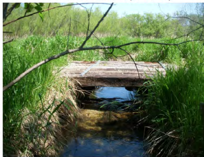
23- PRIVATE BRIDGE 6 PEWAUKEE RIVER (RM 9.40)
