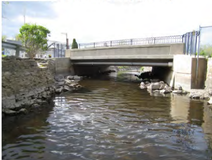
10- OAKTON AVENUE PEWAUKEE RIVER (RM 6.55)
