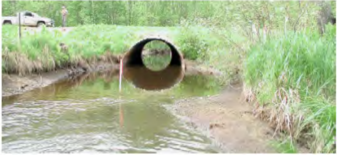
Undersized culvert.
