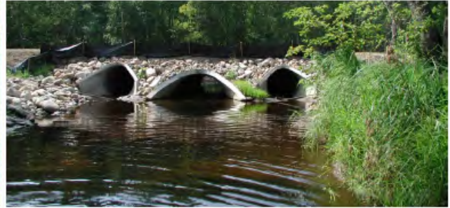
Properly sized and placed culverts.
