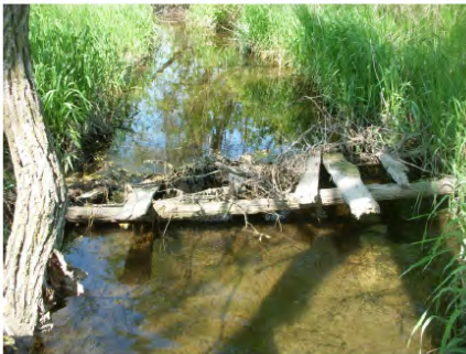
19- PRIVATE BRIDGE 4 PEWAUKEE RIVER (RM 8.65)
