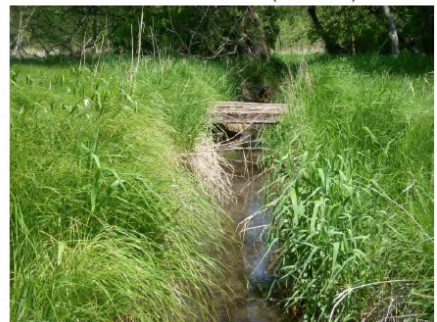
24- PRIVATE BRIDGE 7 PEWAUKEE RIVER (RM 9.55)
