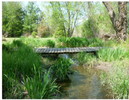
17- PRIVATE BRIDGE 3 PEWAUKEE RIVER (RM 8.62)
