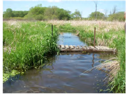
15- PRIVATE BRIDGE 1 PEWAUKEE RIVER (RM 8.12)
