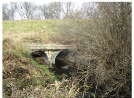
42- CTH KF (RYAN ROAD) COCO CREEK TRIBUTARY (RM 1.34)
