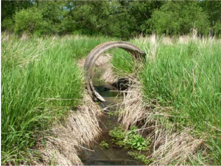
25- PRIVATE CULVERT 1 PEWAUKEE RIVER (RM 9.59 )
