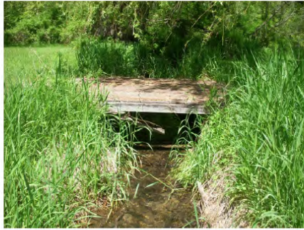
26-PRIVATE BRIDGE 8 PEWAUKEE RIVER (RM 9.63)
