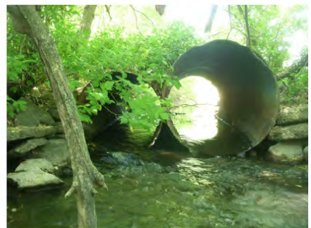
36- PRIVATE CULVERTS COCO CREEK (RM 0.81)
