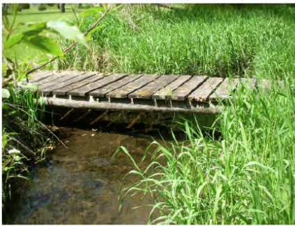
16-PRIVATE BRIDGE 2 PEWAUKEE RIVER (RM 8.57)
