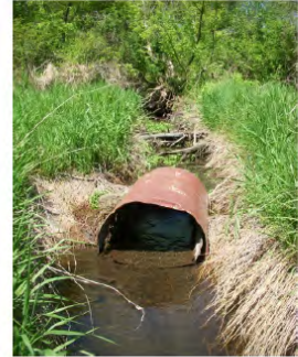
27- PRIVATE CULVERT 2 PEWAUKEE RIVER (RM 9.79)
