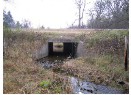
39- CTH JK (LISBON AVENUE) COCO CREEK (RM 3.20)
