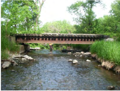
1- ABANDONED RAILROAD PEWAUKEE RIVER (RM 0.05)
