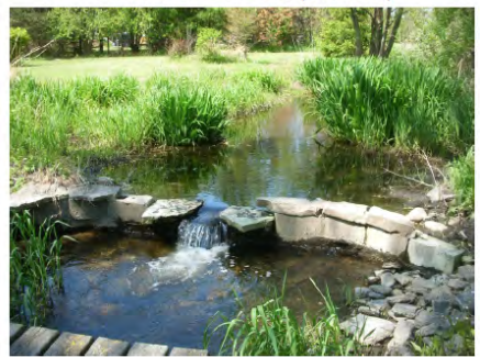
18- PRIVATE DROP STRUCTURE PEWAUKEE RIVER (RM 8.62)
