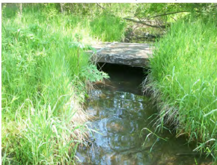
22- PRIVATE BRIDGE 5 PEWAUKEE RIVER (RM 9.29)
