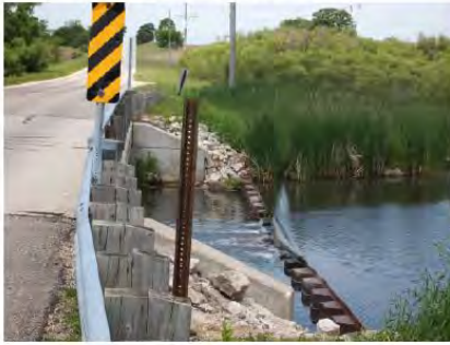
1- MOUND ROAD AND WEIR JACKSON CREEK (RM 1.9)
