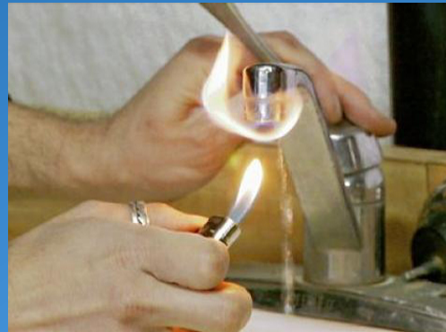
Contamination/Loss of Water Supply
