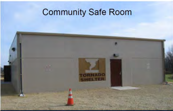
Community safe rooms built to FEMA-361 standards can withstand winds up to 250 MPH. Image from Town of Dunn, WI
