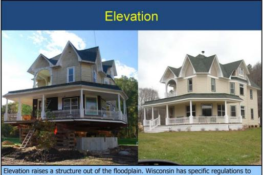
Elevation raises a structure out of the floodplain. Wisconsin has specific regulations to follow with elevation projects. See DNR for more information.
