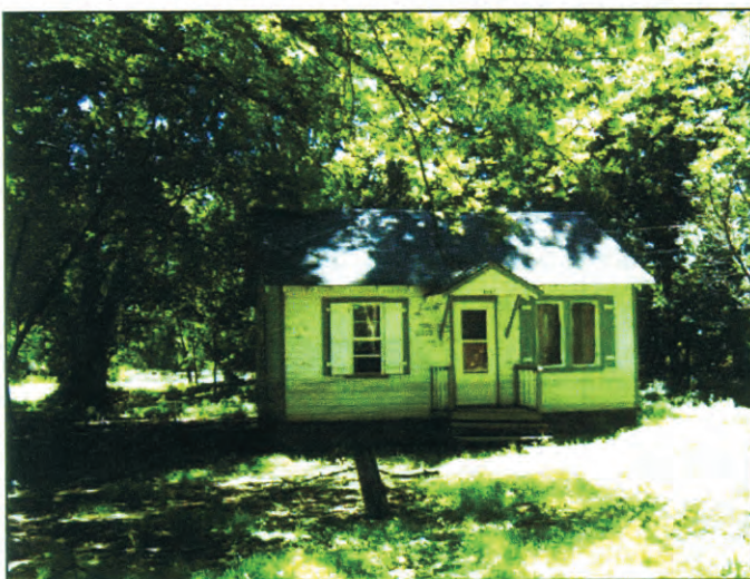
This small house, formerly a vacation cottage next to the Fox River, is one that's been purchased as part of the Fox River Flood Mitigation Project. It will be demolished and the land returned to nature. Photo taken 8/7/08: Barbara Ellis, FEMA
